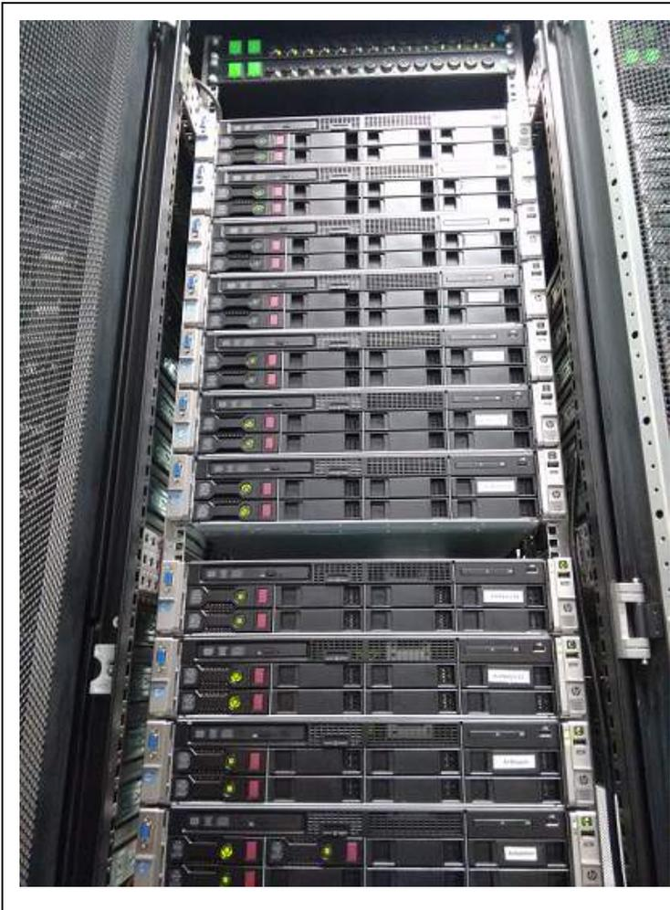
**One of the Cabinets hosting Actus recorders. Every recorder encodes 20 to 30 SD and HD channels and stores proxy files before pushing them to the central storage.**
